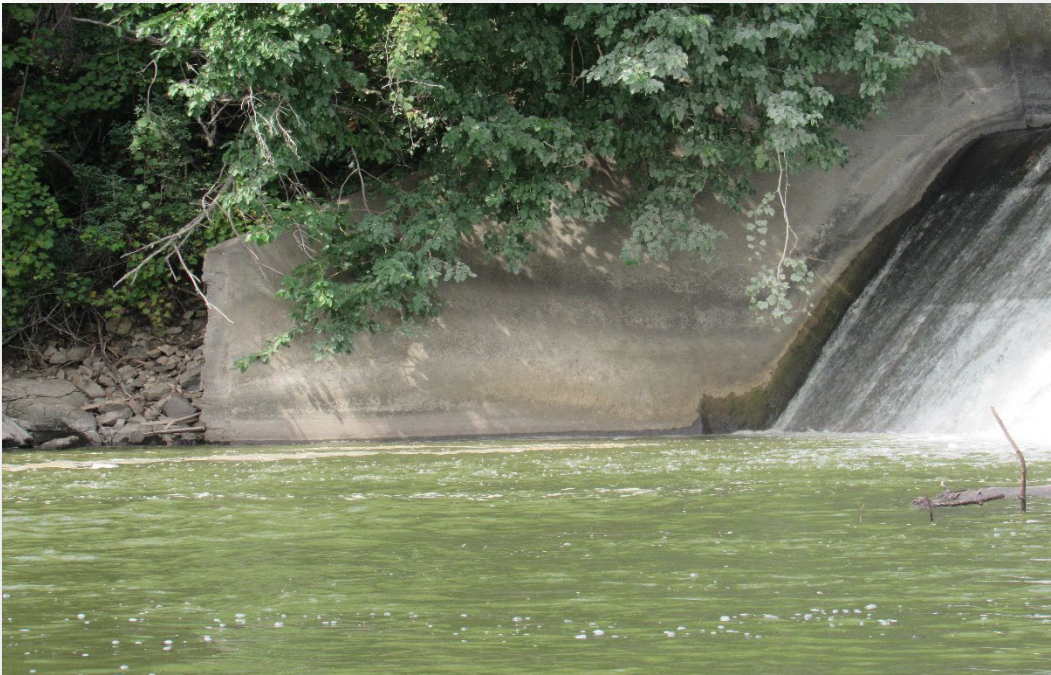
Figure 58 – Downstream, West Wingwall
