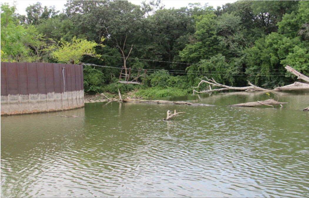
Figure 28 – Upstream, Spillway 3: Timber Debris Accumulation
