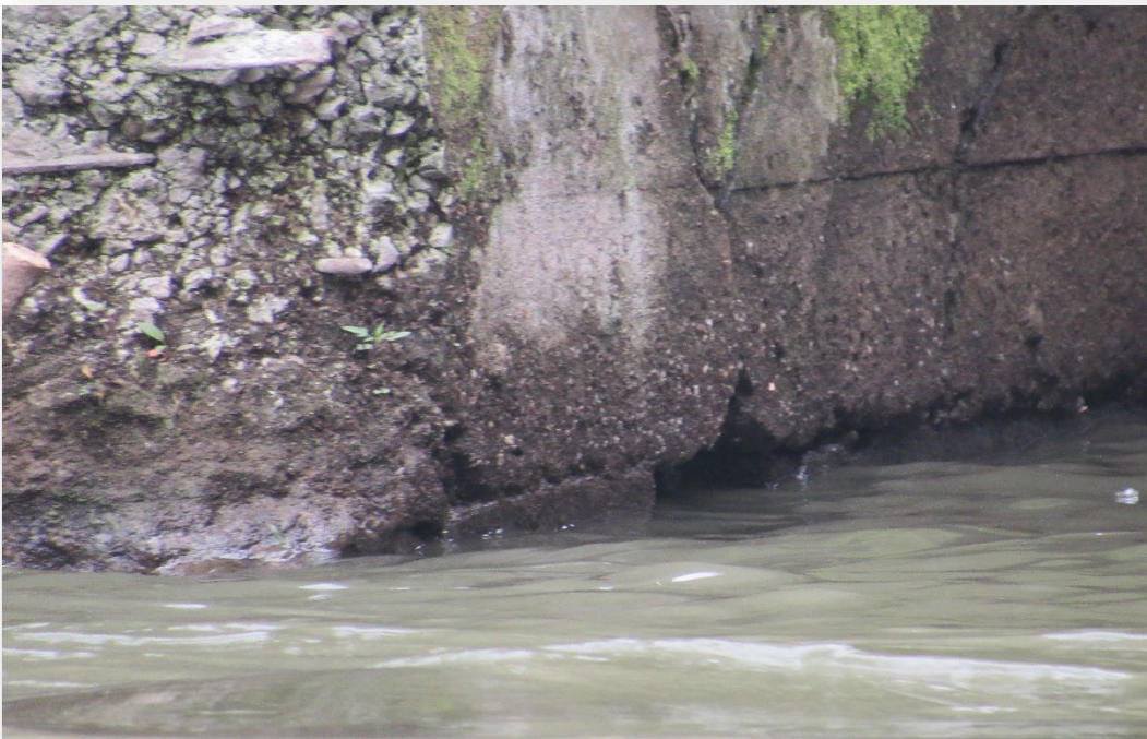
Figure 45 – Downstream, Control Gate West Pier
