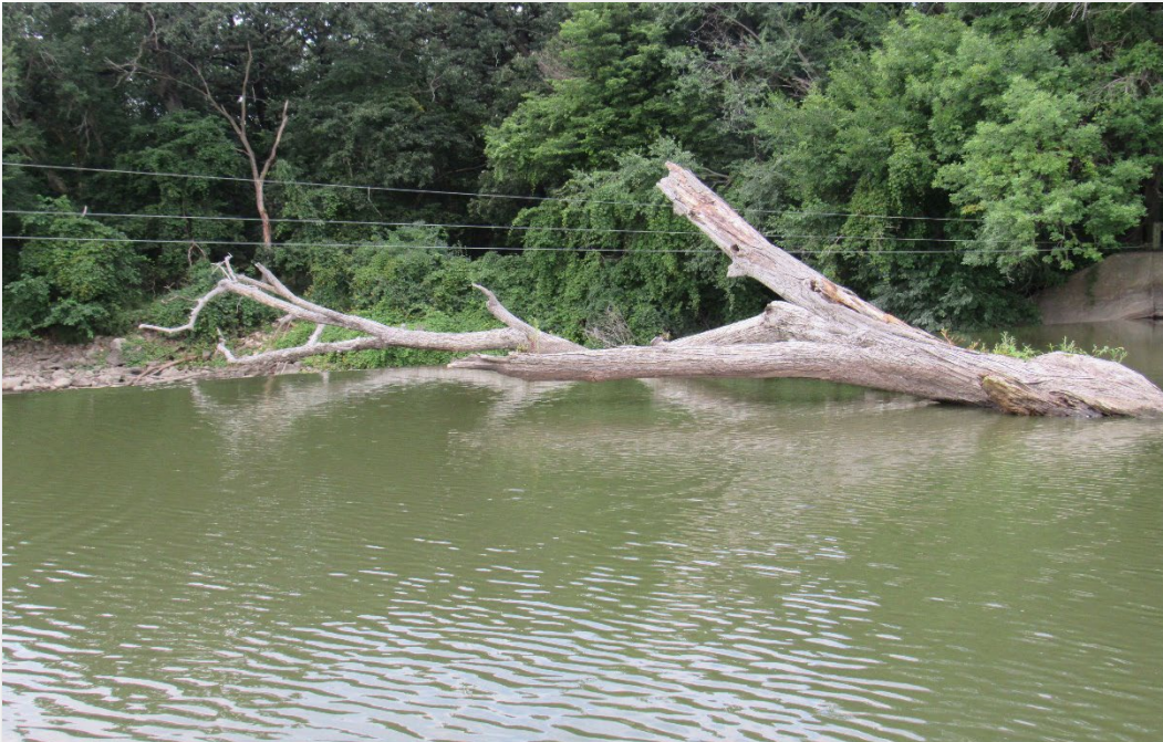
Figure 29 – Upstream, Spillway 3: Timber Debris Accumulation
