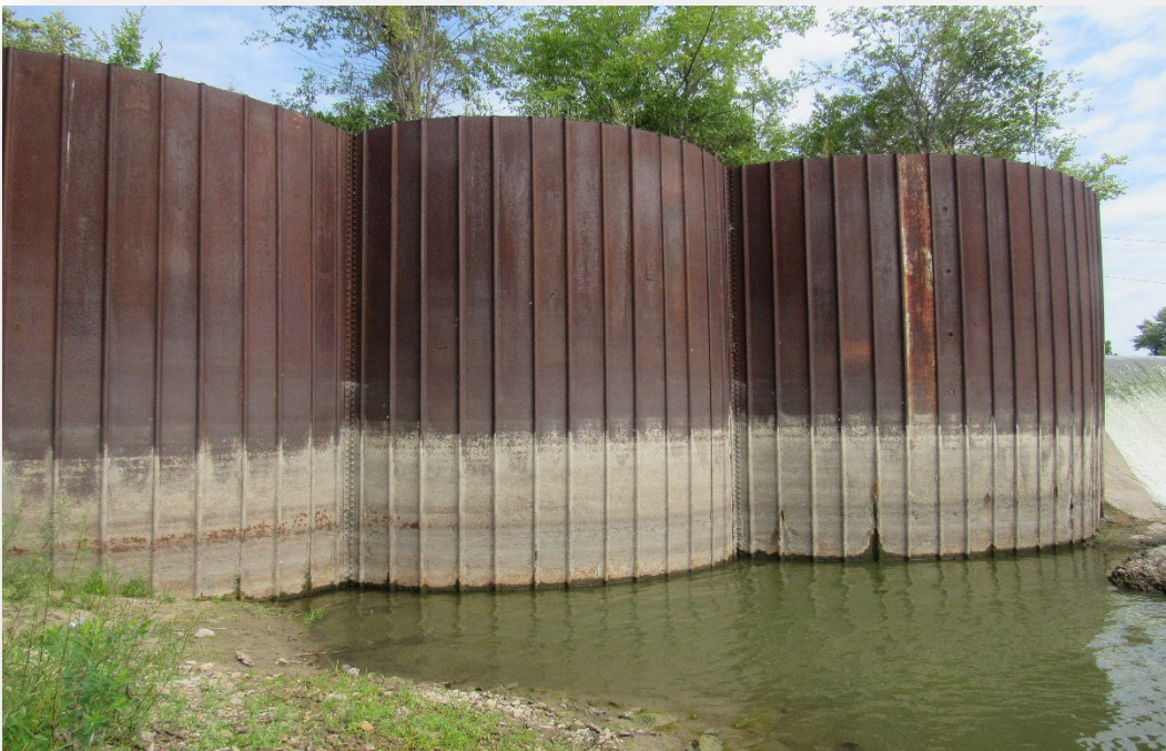
Figure 53 – Downstream, Cell Section
