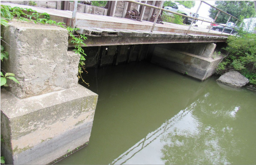
Figure 32 – Downstream, Eastern Bypass
