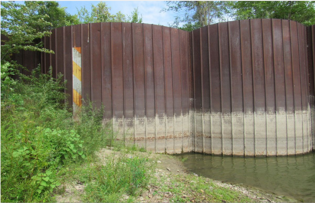
Figure 54 – Downstream, Cell Section
