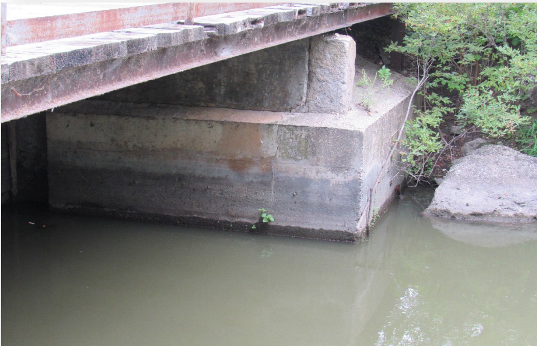
Figure 33 – Downstream, Eastern Bypass
