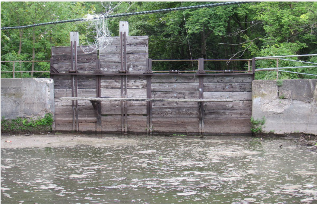
Figure 5 – Upstream, Eastern Bypass: Timber Gate
