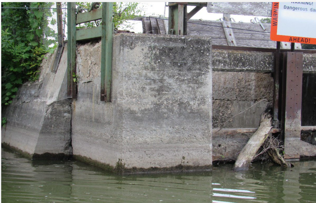
Figure 9 – Upstream, Control Gates
