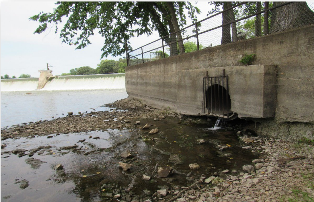
Figure 37 – Downstream, East Wingwall
