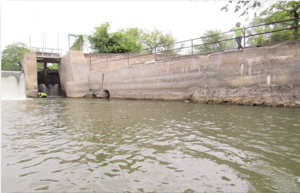
Figure 40 – Downstream, East Wingwall: Overview
