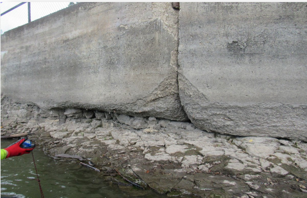
Figure 39 – Downstream, East Wingwall: Scale Band
