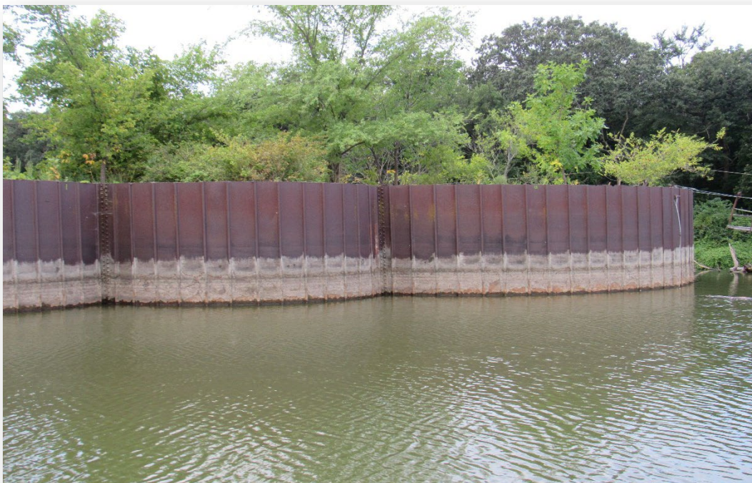
Figure 25 – Upstream, Cell Section
