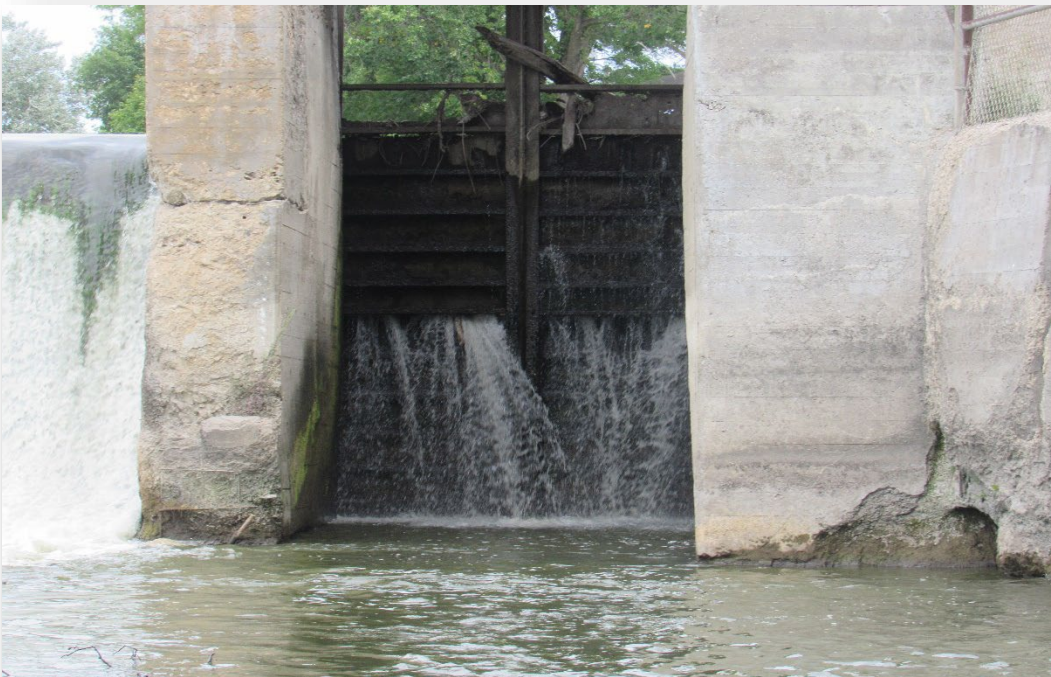
Figure 43 – Downstream, East Wingwall and Control Gates
