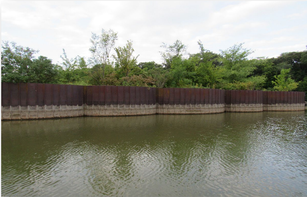
Figure 24 – Upstream, Cell Section
