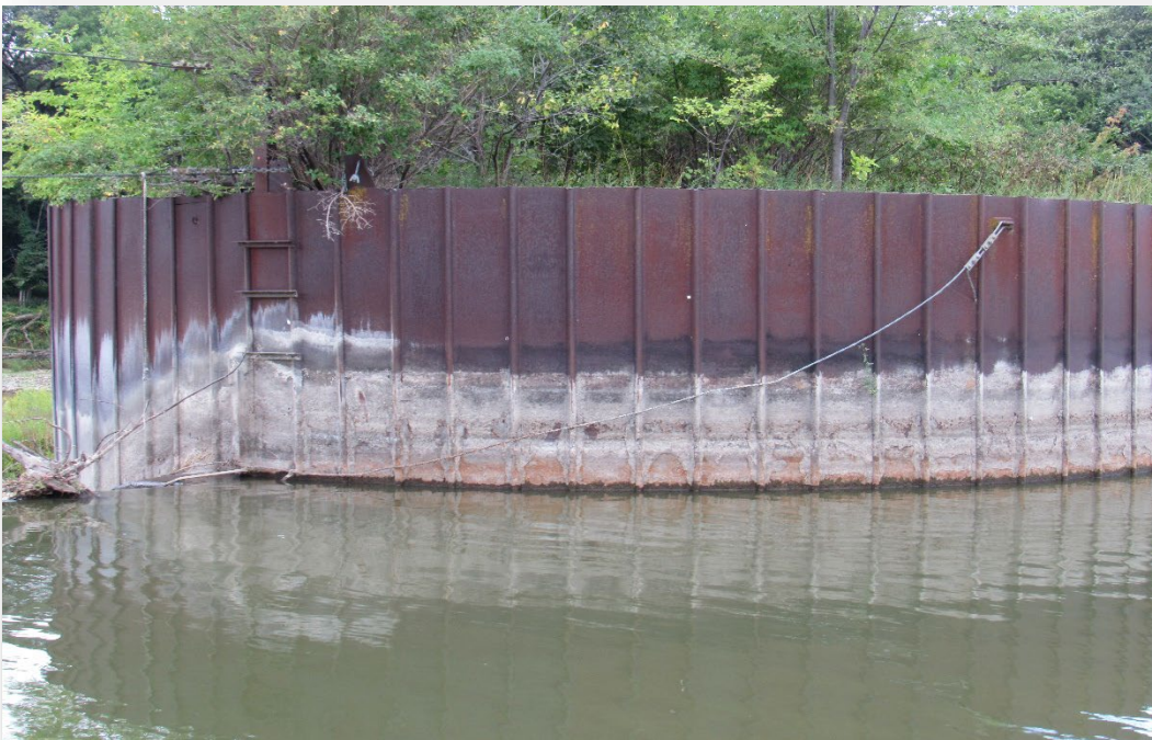
Figure 21 – Upstream, Cell Section
