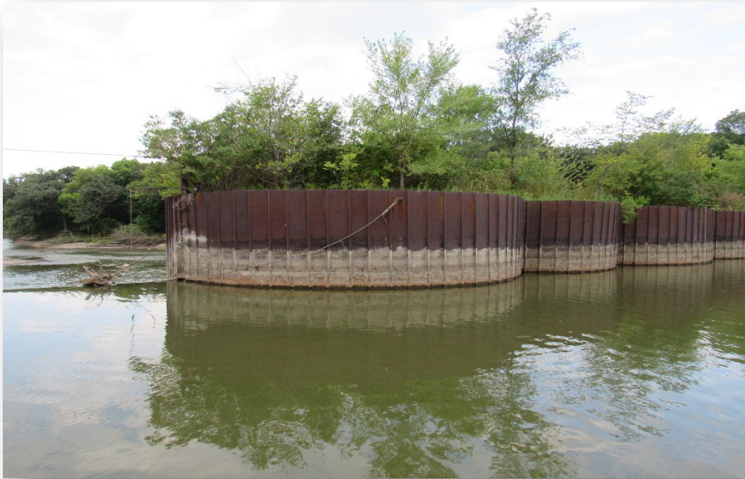
Figure 22 – Upstream, Cell Section
