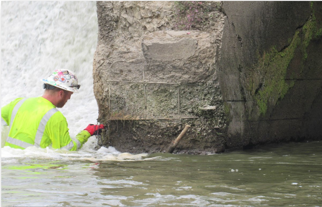
Figure 46 – Downstream, Control Gate West Pier:
