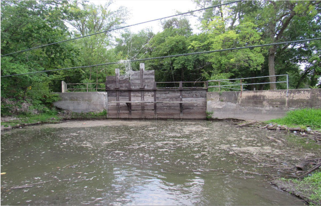
Figure 2 – Upstream, Eastern Bypass
