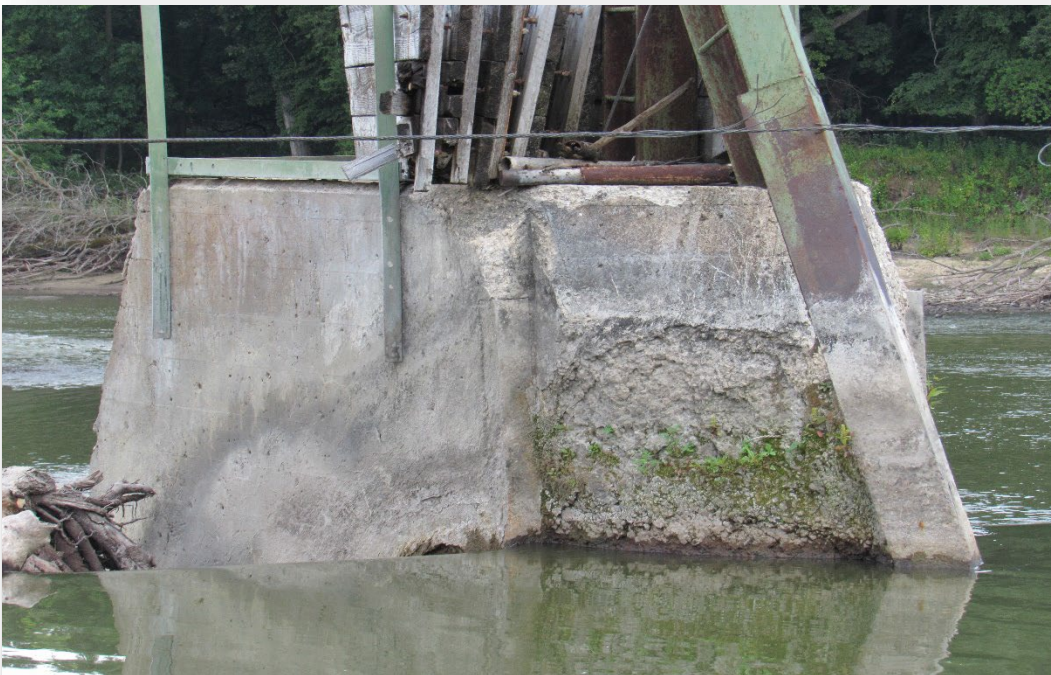
Figure 17 – Upstream, Spillway: Center Pier
