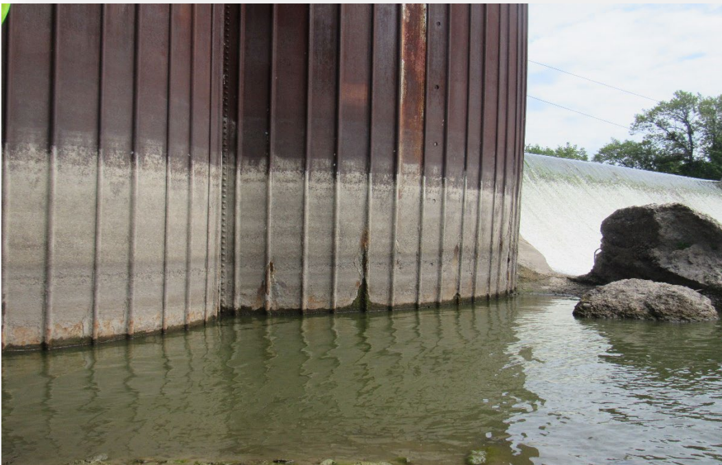
Figure 51 – Downstream, Cell Section
