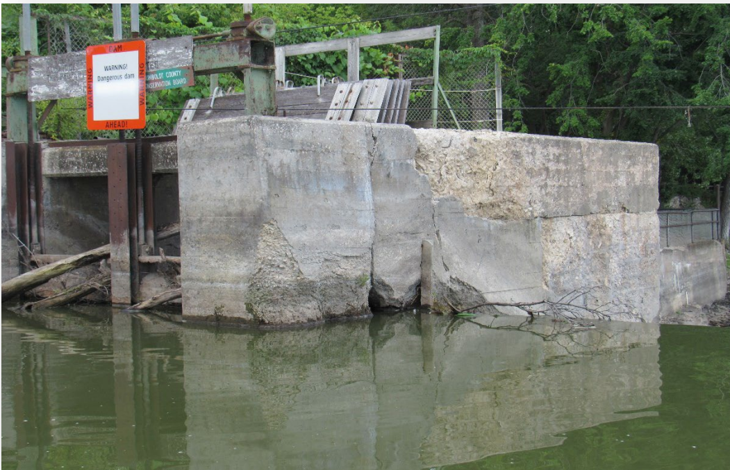
Figure 15 – Upstream, Control Gates West Pier: Overall Condition
