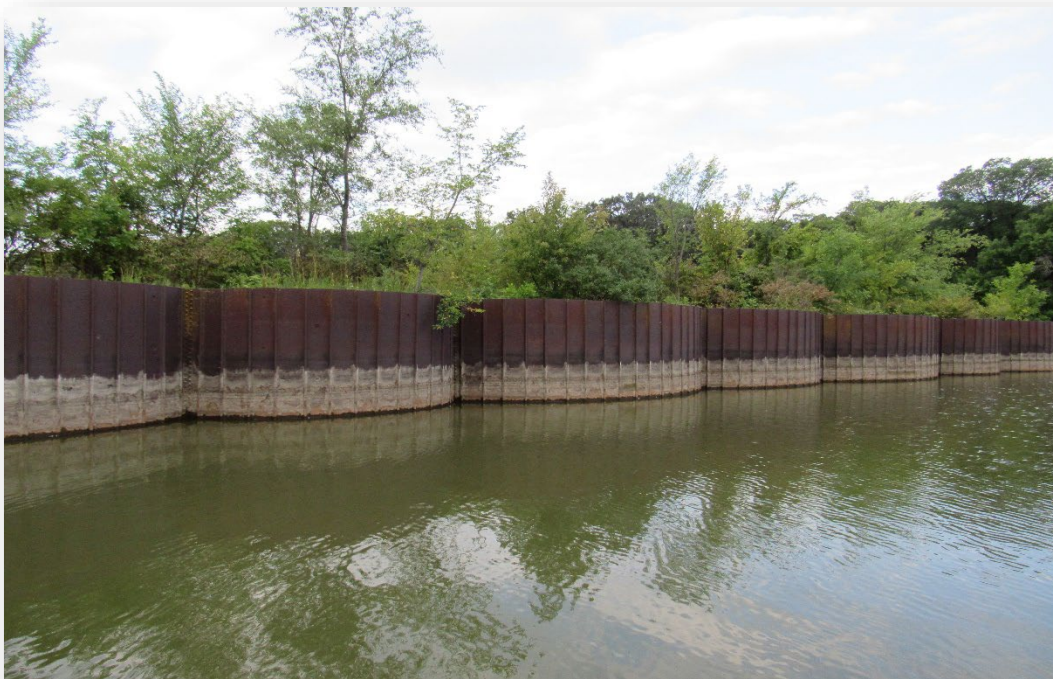
Figure 23 – Upstream, Cell Section
