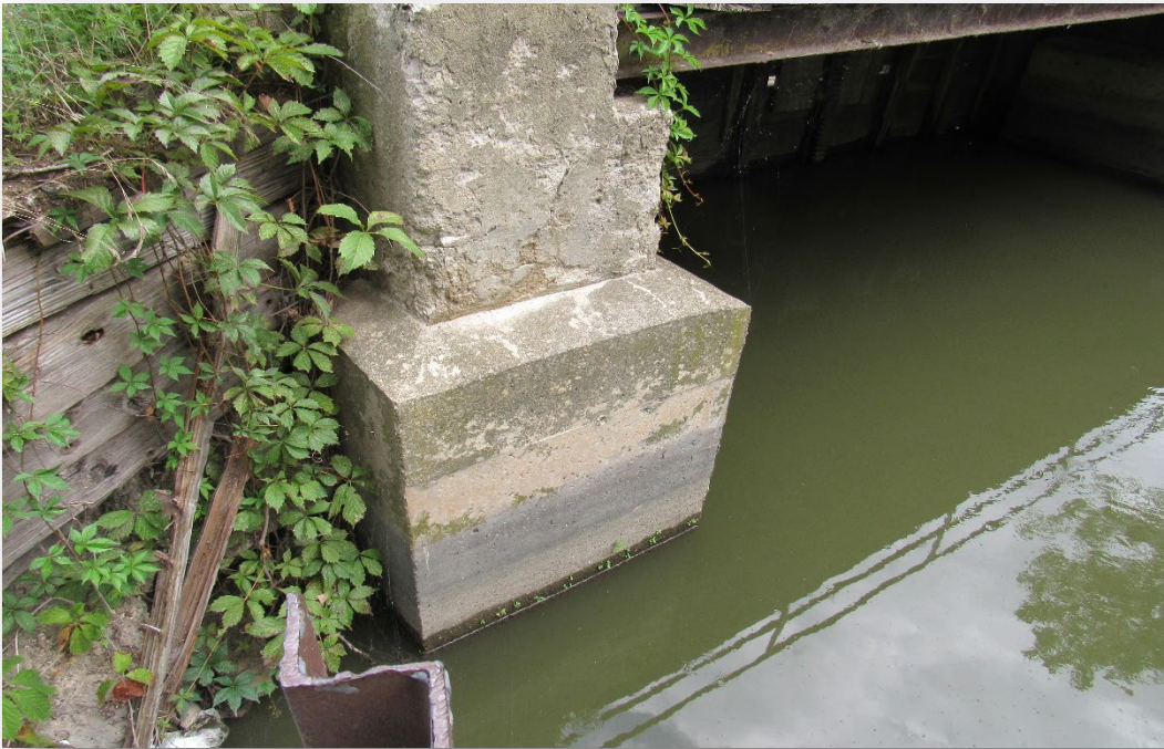
Figure 34 – Downstream, Eastern Bypass
