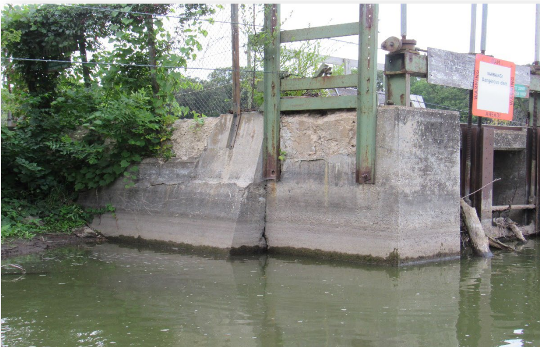
Figure 7 – Upstream, Control Gates East Pier
