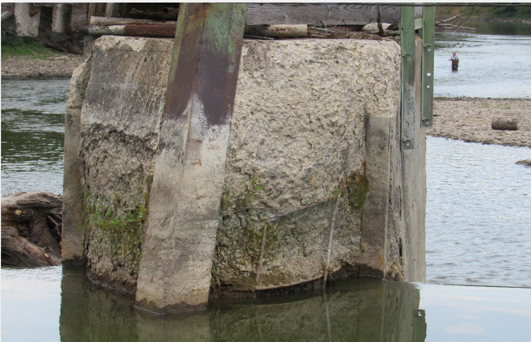
Figure 19 – Upstream, Spillway: Center Pier
