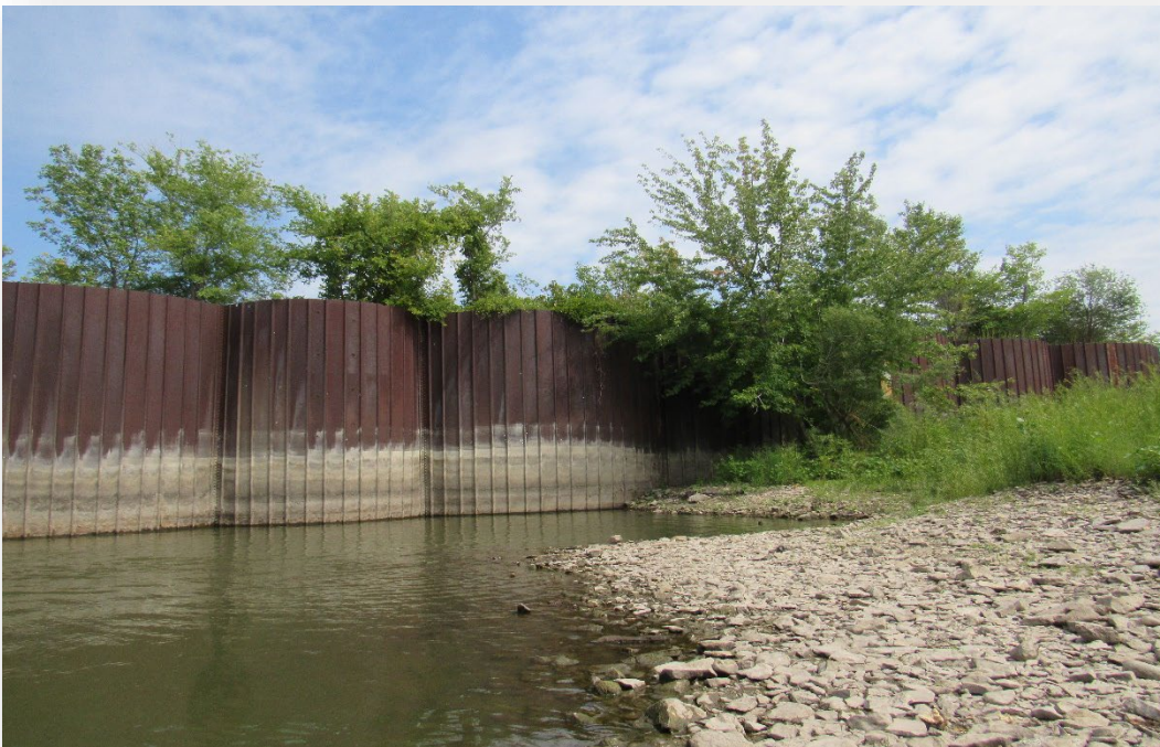
Figure 55 – Downstream, Cell Section
