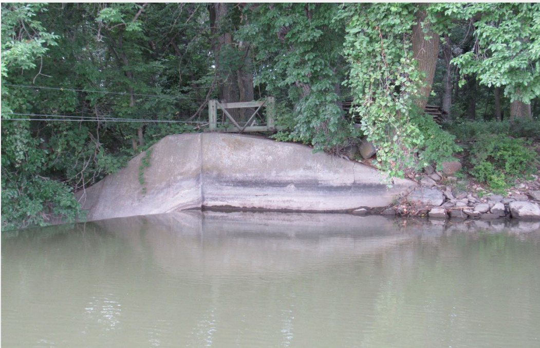
Figure 31 – Upstream, West Wingwall
