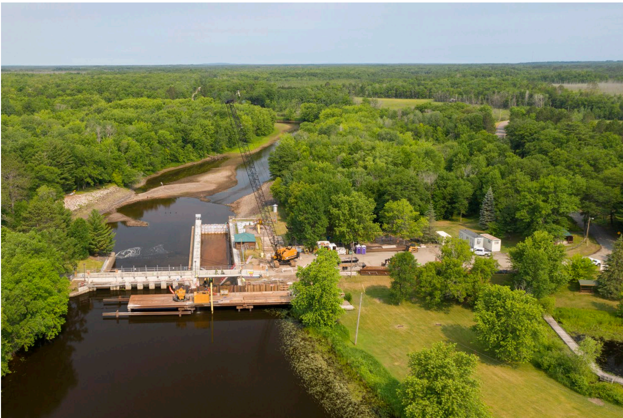
Temporary access trestle example
