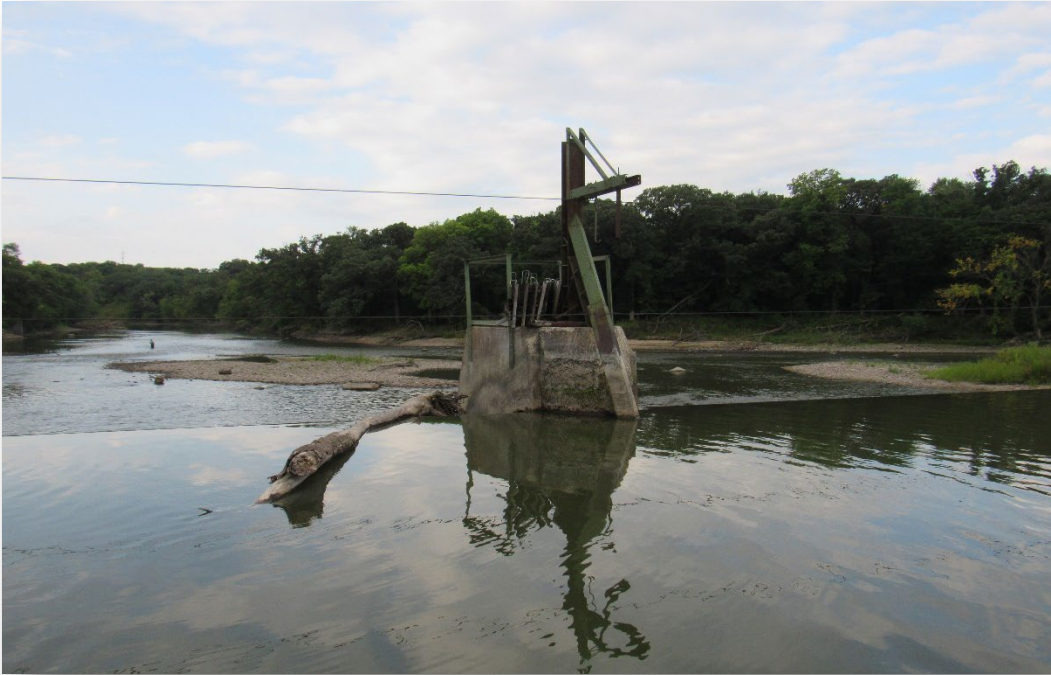
Figure 18 – Upstream, Spillway: Center Pier
