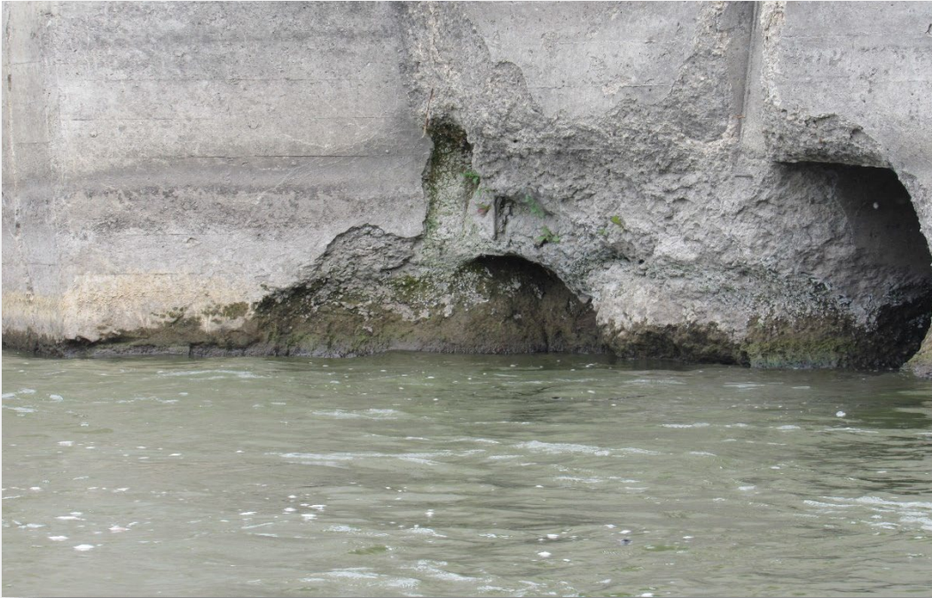
Figure 42 – Downstream, East Wingwall
