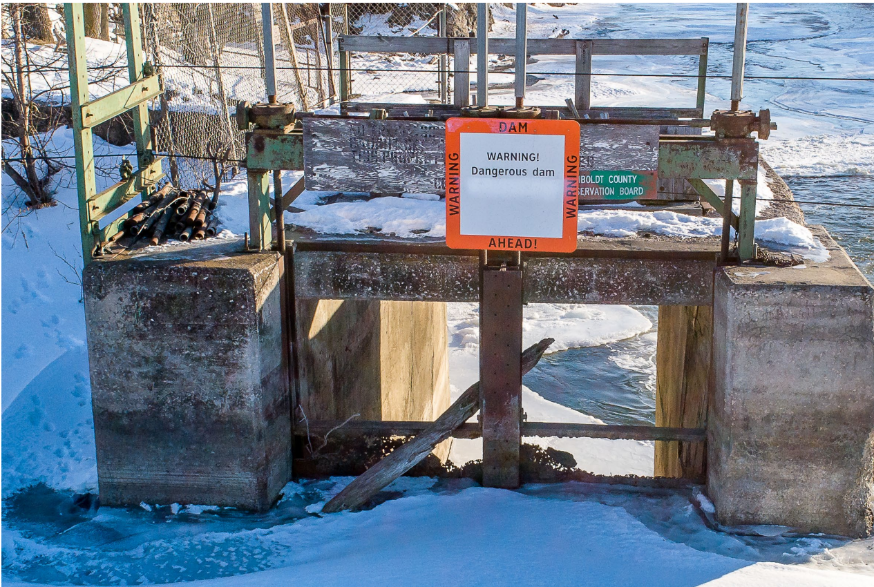
Recent conditions of the existing slide gate.
